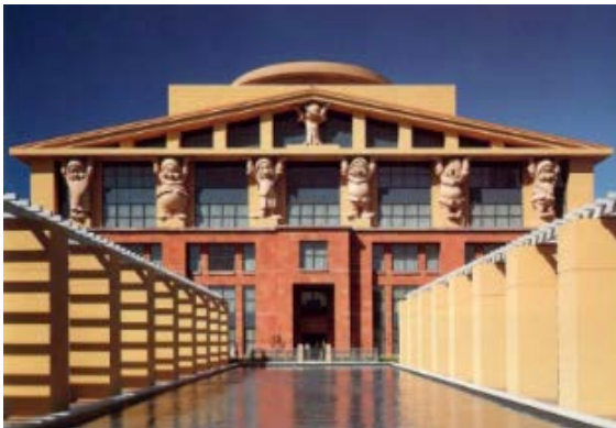
Team Disney Building, 1989-1990
